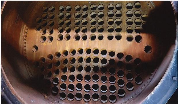
Original 1924 Kewanee Boiler still sits in boiler room ground level of our Cathedral. Similar to coal fired steam locomotive boilers this unit has now been replaced with a natural gas unit utilizing radiator heating throughout your building.
